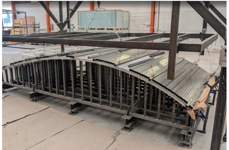
Building the cavity of the panel mould at FERRUM. (Credit: FERRUM)
