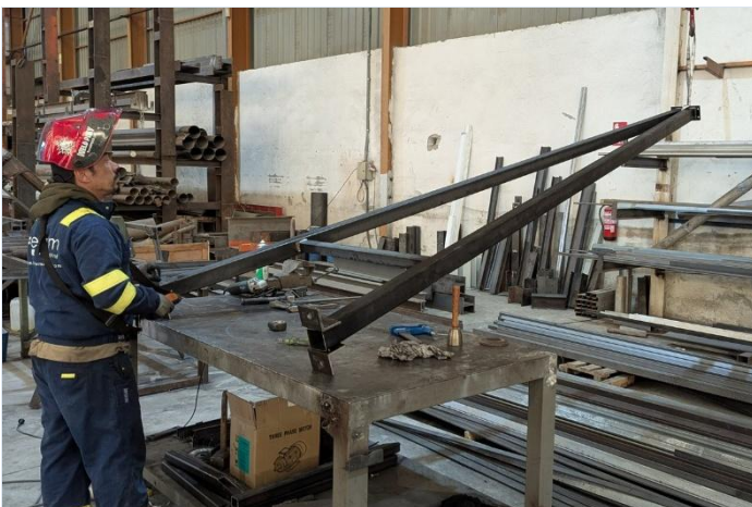
Steel structure and pylons in fabrication at FERRUM.
