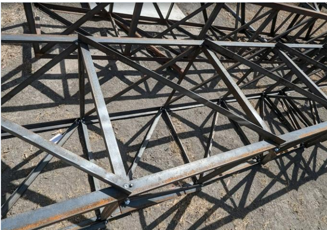
Triangular truss frames and torque boxes fabricated at FERRUM.
